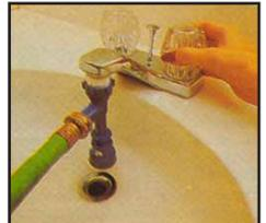
D. Once water is flowing into the bed for a few seconds, turn the "bell valve" to the "down" position, leaving the water flowing full blast. The water from your faucet flowing through your drain pump will suck the water out of your bed. This will take one or two hours depending on water pressure. Do not allow air to get in the hose.
