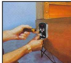
**C.** Run the thermostat control's sensor cable through the corner hole inside the frame onto the deck. The sensor cord should be positioned midway between the frame and the heating pad, preferably twelve inches away from the heating pad.
